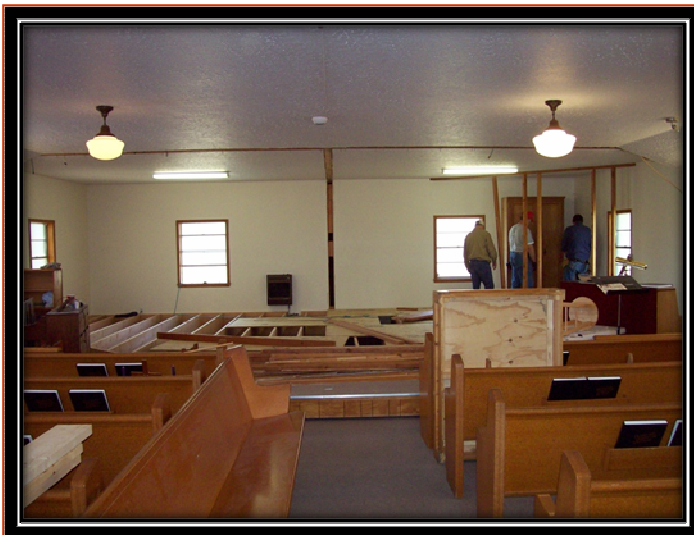
Butch Chappell , Alvin Lievsay, and Ron Woollen framing storage areas in the newly expanded chancel. The older pews, made of a compressed particle board material, can be seen in the foreground.
